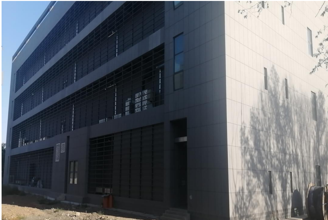
A data center in Urumqi, Xinjiang Province, China
