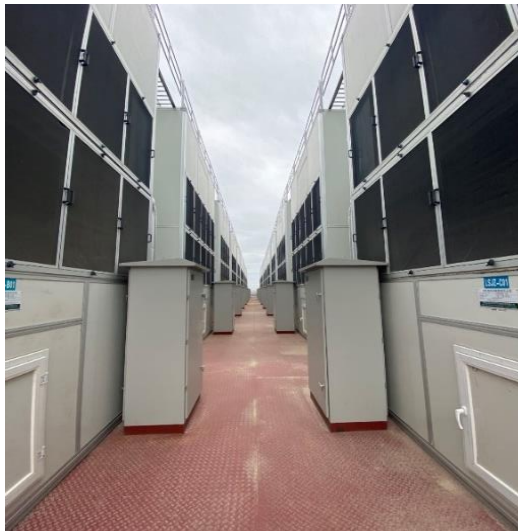
IEC water chillers on the roof
